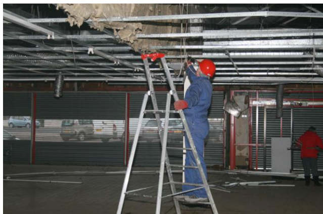
Making a Start on Removing the Ceiling Grid
